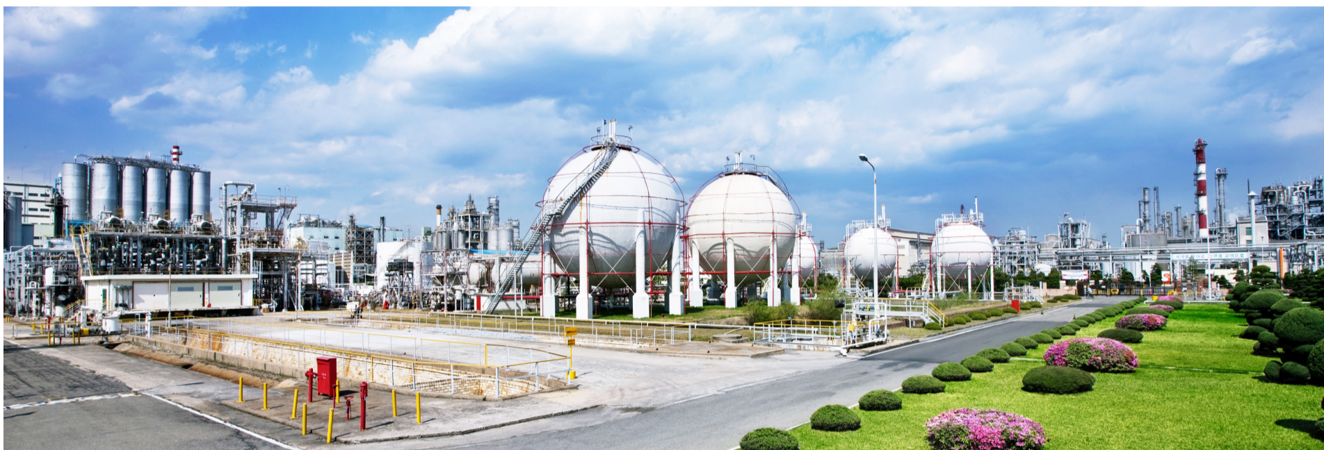
Hanwha Chemical Ulsan Plant
