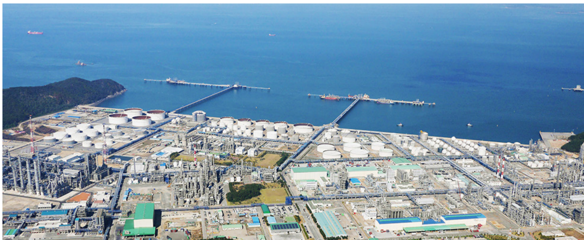
Hanwha Total Petrochemical's Daesan Production Facility, the site of the new 400,000-ton PE expansion plant
