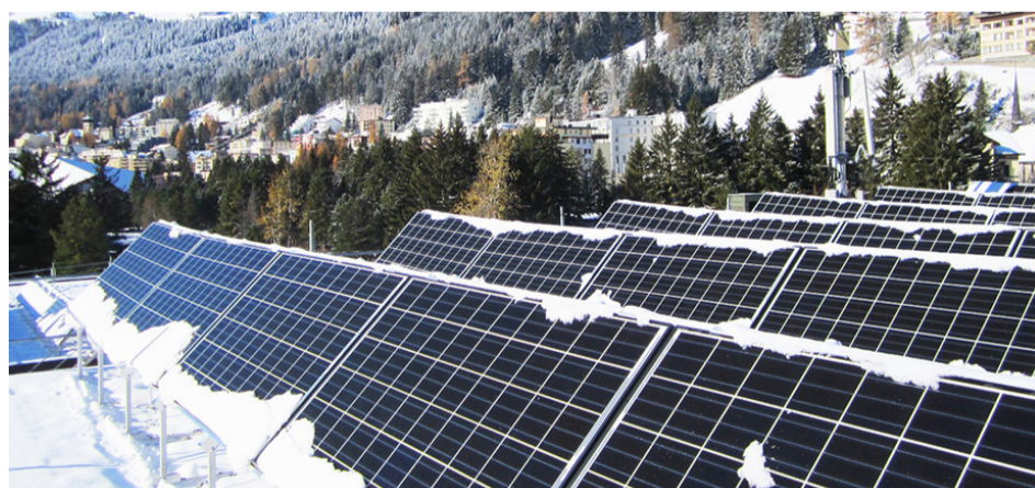
Hanwha Q CELLS' solar modules on the roof of the Davos Congress Centre
