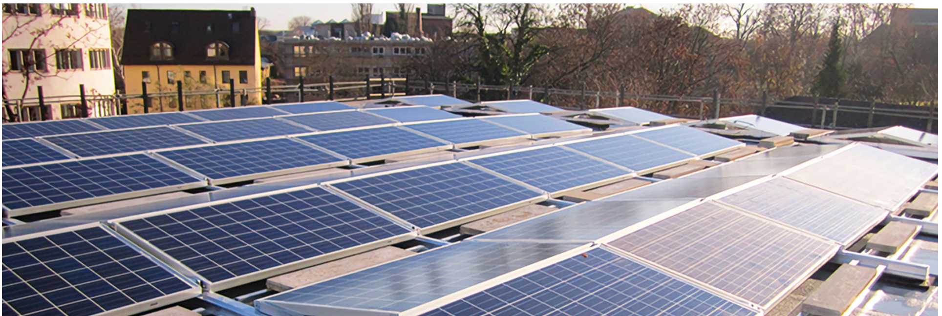
Hanwha Q CELLS' Solar panels installed onto the roof in downtown Frankfurt, Germany
