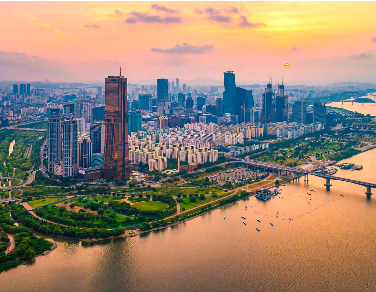
63 Hanwha Life building
