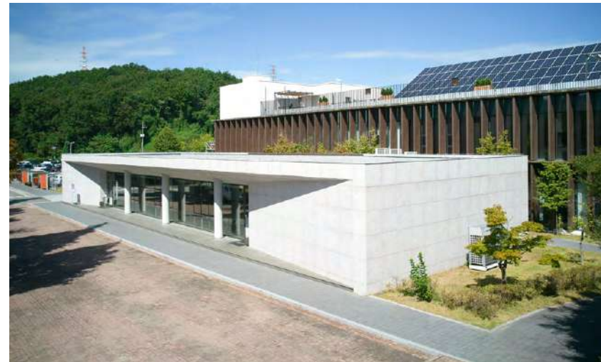
Hanwha Advanced Materials manufacturing facility
